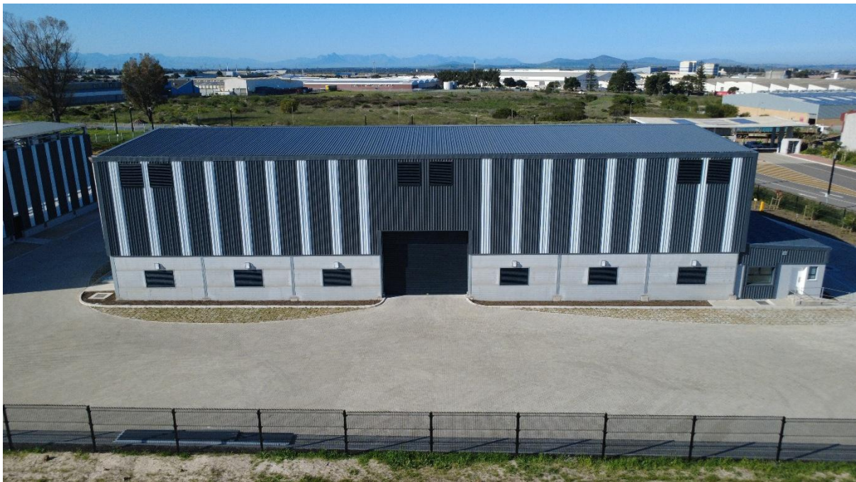
Figure 2: Quantum V3 Facility Main Building to house the Solar & Battery Solution
