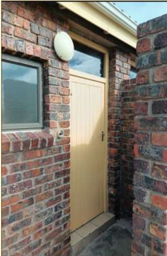
Wooden doors, frames and top window to be removed
