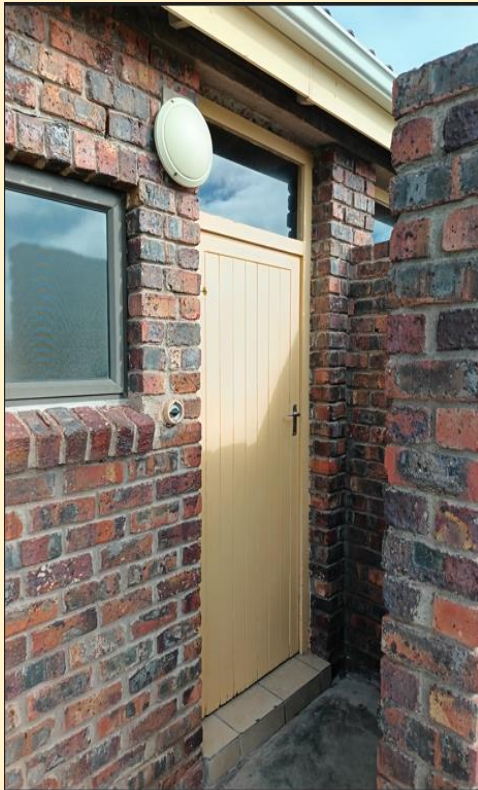
Wooden doors , frames and top window to be removed
