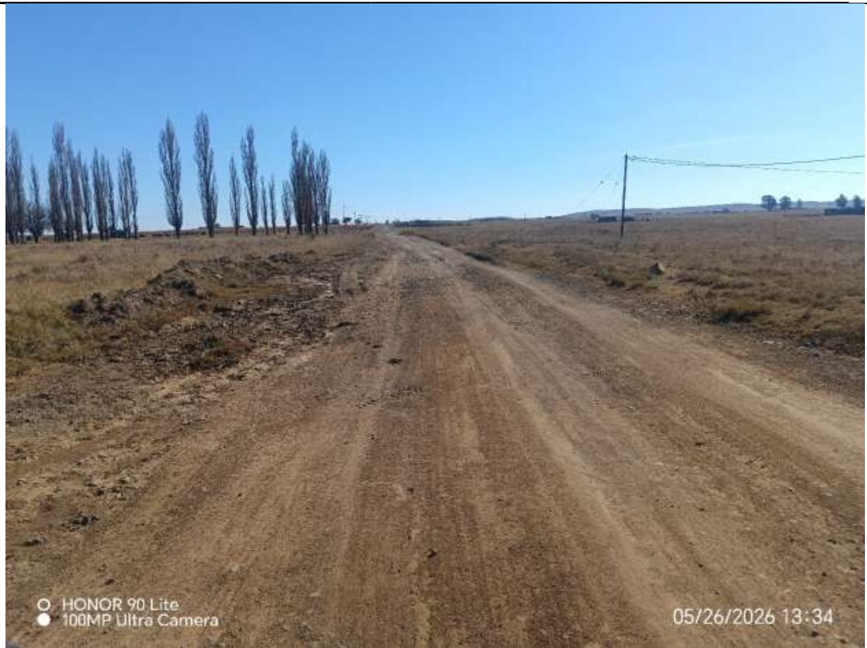
Existing gravel road 2
