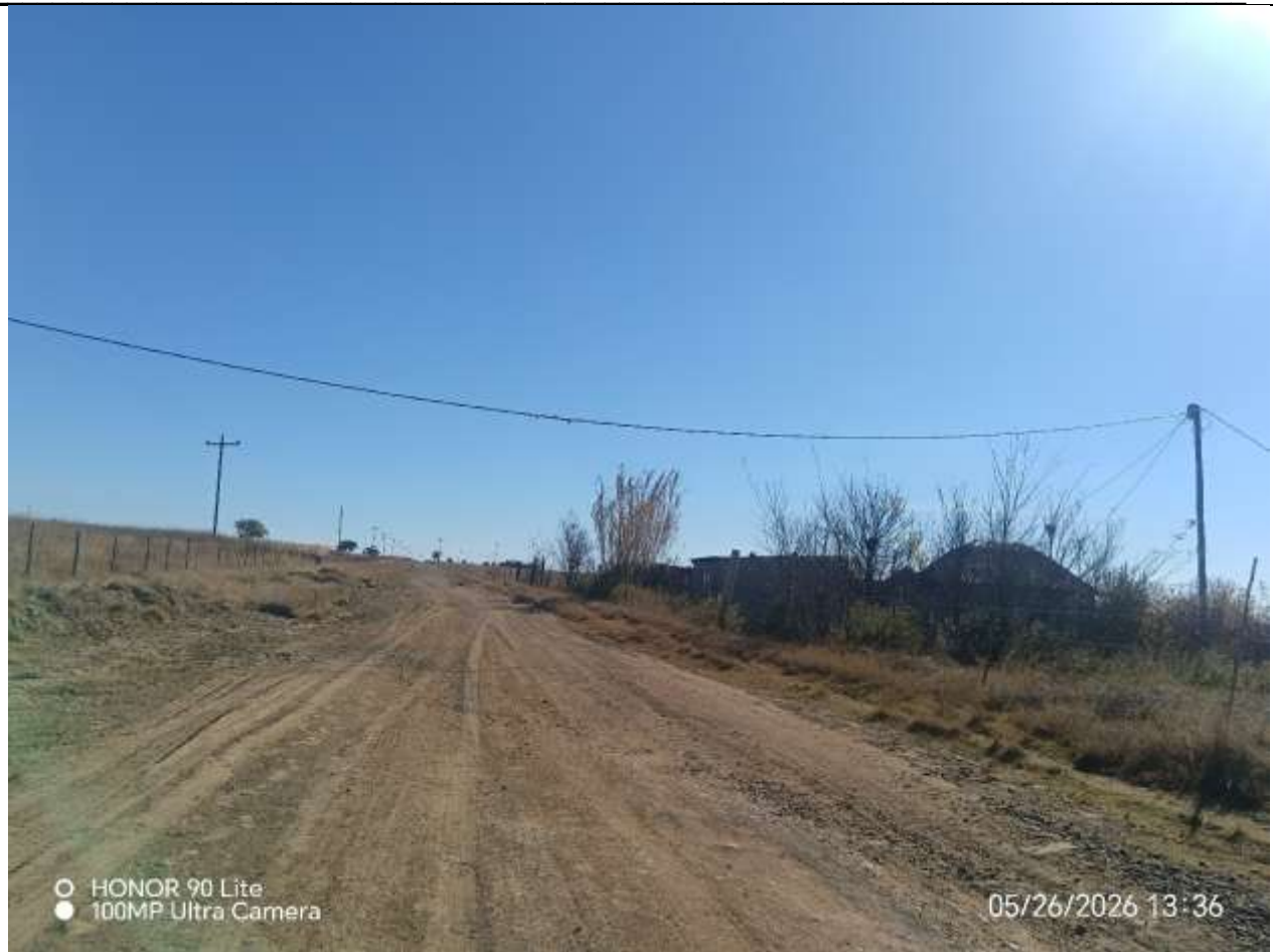
End of Road 2
