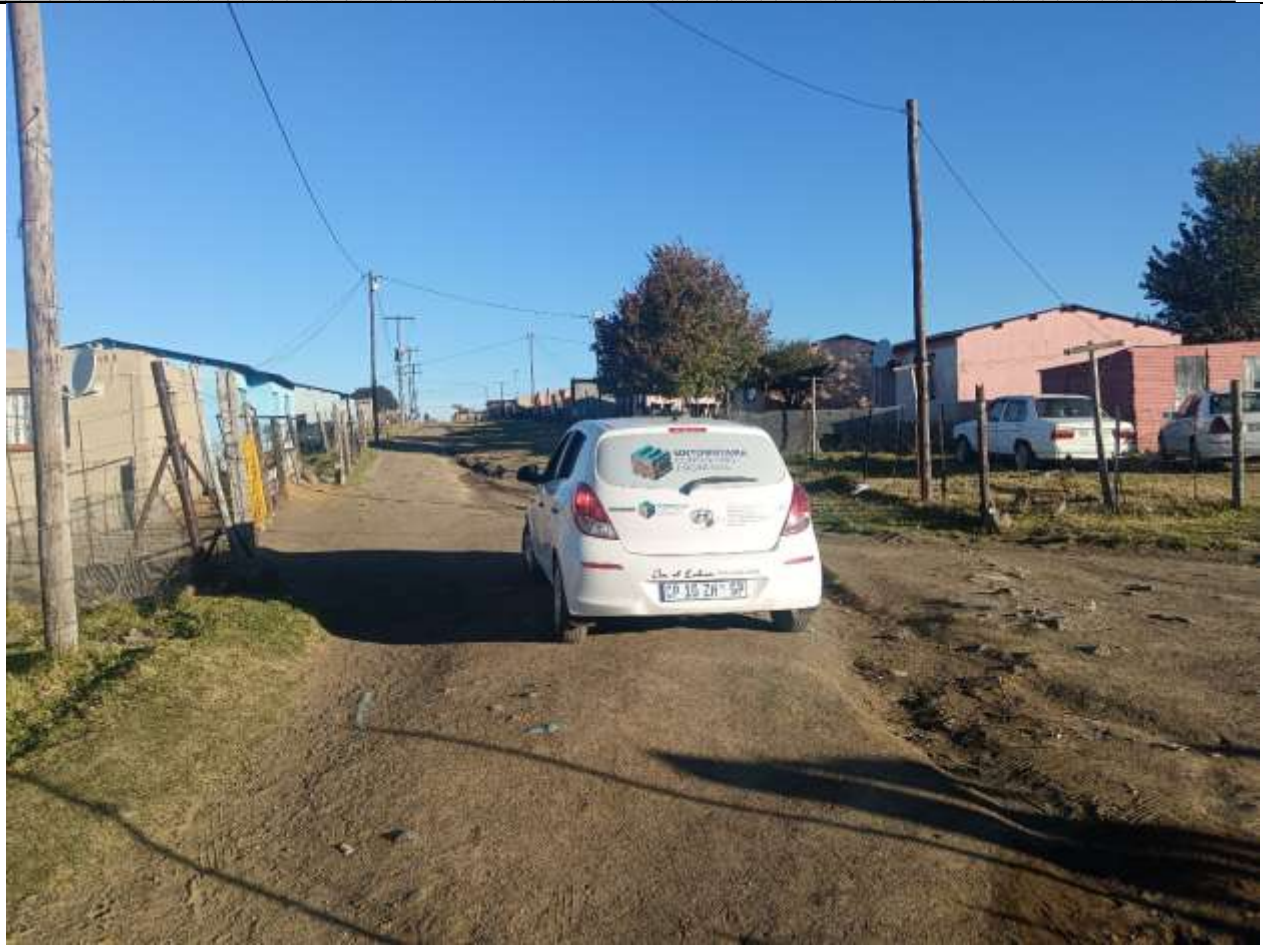
End of road 4 ward 7
