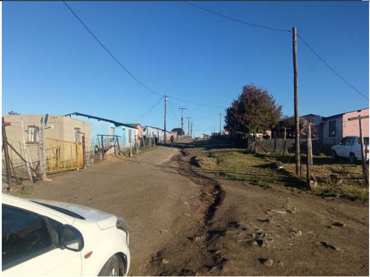
Road 4 Wrad 7: Erosion due to uncontrolled stormwater
