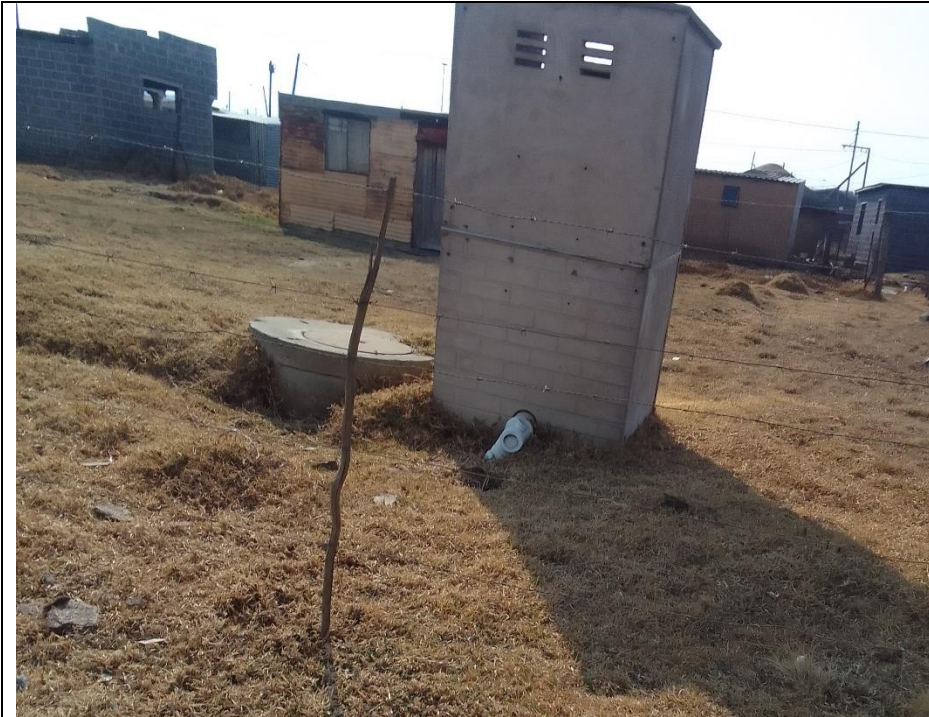
Figure 3: Existing Manhole, toilet and house connection in Ward 01
