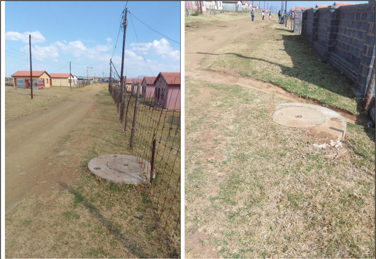
Figure 8: Existing Manhole along the street in Ward 02
