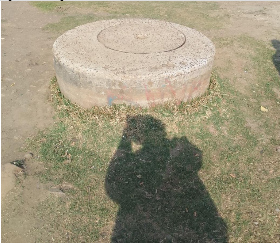
Figure 4: Existing Manhole along the street in Ward 01
